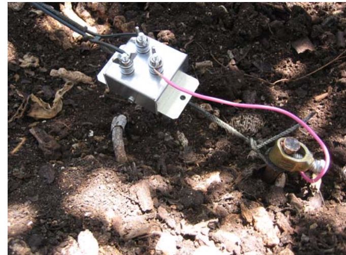
Figure 4: Photographs of the near and far end terminations of a Ducie Island two-wire beverage.
